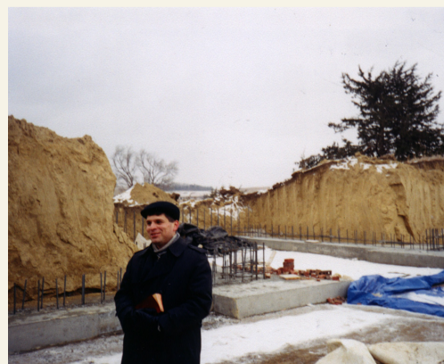
Visitor Center foundations
